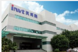
Shenzhen Fuyong Industrial Park
